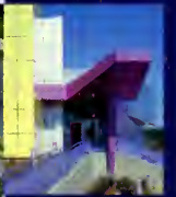
EXTRADE REGIONAL OPERATIONS CENTER ATLANTA, GEORGIA
